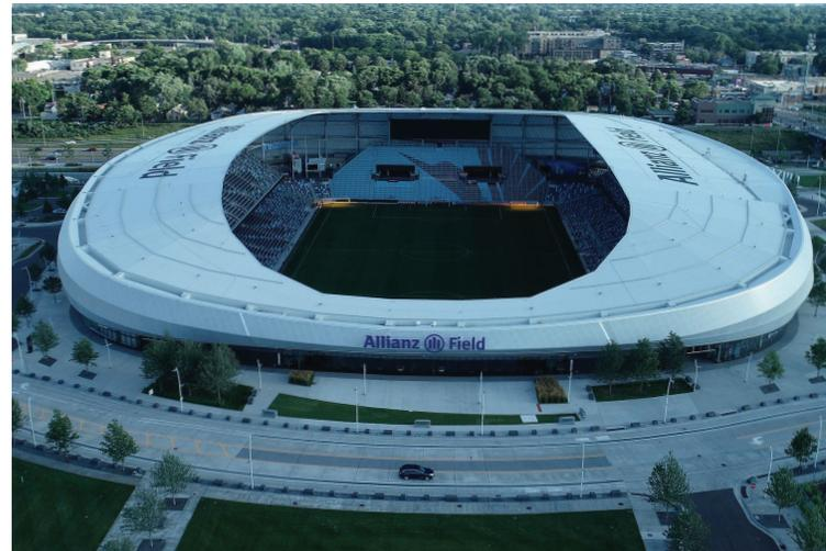
Today, foot traffic on the canopy roof is limited to use of the safety line system for maintenance of the roofing, gutter system, and drains.
