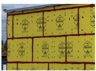
the gypsum core, beneath the fiberglass mat, to create a consistent, performance-tested WRB-AB. No building wrap, fluid-applied membranes or peel-and-stick membranes are required. Bill Perry of Tiger Construction appreciated the elimination of a step in the process, "The Z girts to support the cladding did not have to be
