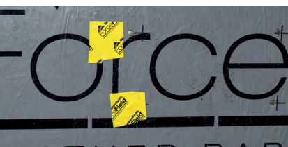
04 OVERDRIVEN FASTENER WITH TAPE TREATMENT
