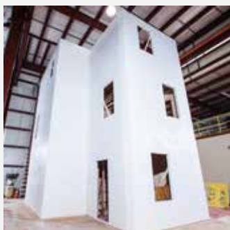
Trial 2: Fluid-Applied Membrane WRB-AB System
