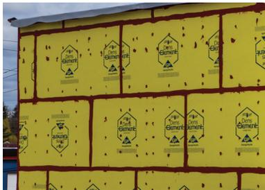
the gypsum core, beneath the fiberglass mat, to create a consistent, performance-tested WRB-AB. No building wrap, fluid-applied membranes or peel-and-stick membranes are required. Bill Perry of Tiger Construction appreciated the elimination of a step in the process, “The Z girts to support
