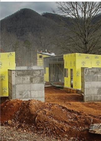
The key to the unique capabilities of the DensElement™ Barrier System lies in a proprietary formulation known as AquaKOR™ Technology which integrates the gypsum core and the fiberglass mat to form a hydrophobic, monolithic surface that blocks bulk water but allows vapor to pass through. Offering optimal performance without the need for an additional WRB-AB means DensElement™ Barrier System can be installed faster and with fewer costs, and using PROSOCO
