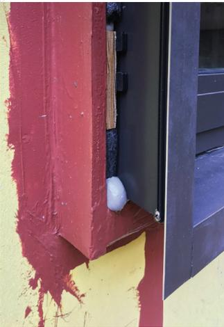
After seeing the DensElement™ Barrier System, with PROSOCO R-Guard® FastFlash® liquid flashing in application, they realized there was a solution that was superior to a traditional self-adhered membrane.
