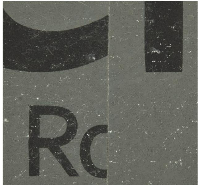
Since the roofing contractor is responsible for the proper installation of roof boards, among many other components, he needs to calculate the amount of expansion that is expected across the range of conditions the roof will experience to allow the materials to expand or contract without affecting roof performance. This can be done by gapping cover boards in the length and width directions. Gapping, however, can be problematic for a number of reasons, such as:
