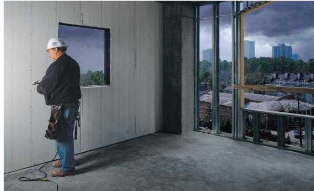
interior panels and DensGlass Shaftliner panels help limit this potentially costly gamble. These products resist damage from humidity and normal weather exposure such as blowing rain because they have fiberglass mats front and back, rather than paper facings. Using moisture-resistant, fiberglass mat gypsum products can improve scheduling accuracy, support shorter construction schedules—and reduce the risk of costly remediation or rip out.
