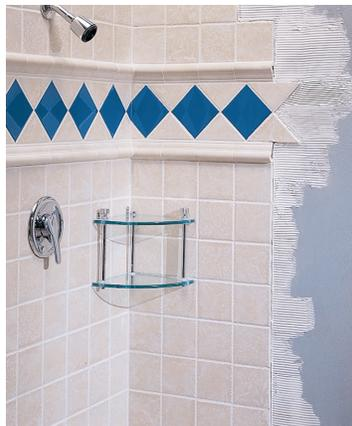
**BACKED UP:** G-P's DensShield is a glass-mat tile backer that has an acrylic coating to prevent moisture from entering the wall cavity.
