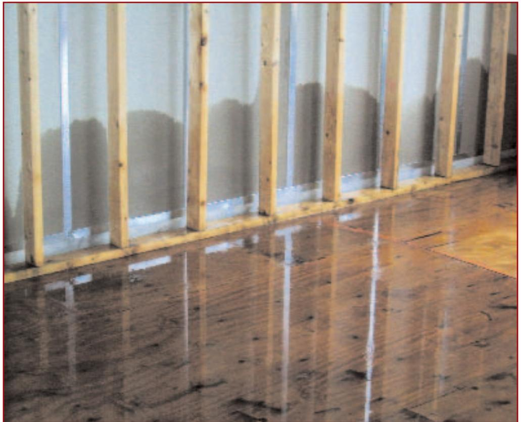
*Water intrusion during construction can wreak havoc on interior drywall, setting the stage for mold contamination.*
