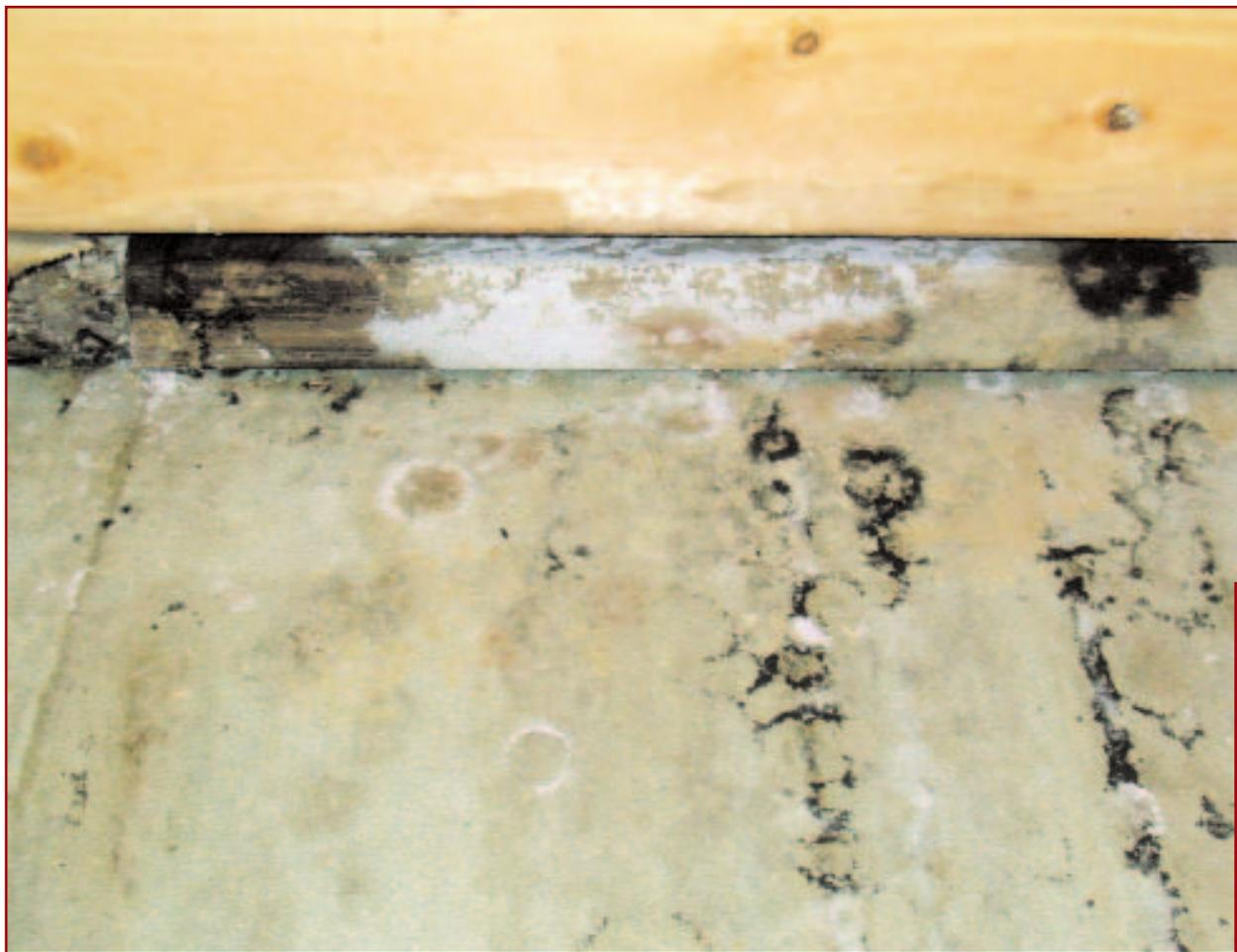
*Moisture and condensation are terrific conditions for mold. Moisture-laden wood wets paper-faced drywall, creating a feast for mold.*
