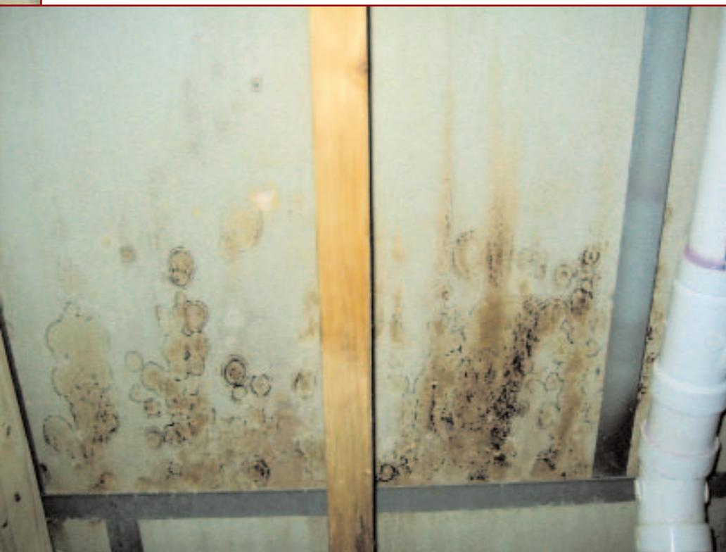
*Leaking pipes and high moisture environments, combined with paper-faced drywall, can turn a recreation room into a mold room.*
