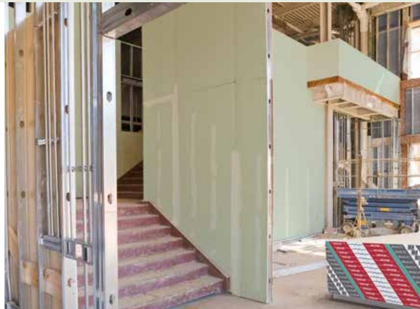
*ToughRock® Fireguard X™ Mold-Guard™ Abuse-Resistant Gypsum Board is a ready-to-finish panel with a smooth, light-colored facer that accepts most types of paints, textures and decorative finishes with no special preparation.*
